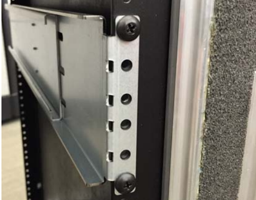
Figure 5. Outer Rack Support attached to the rear-left rack rail
