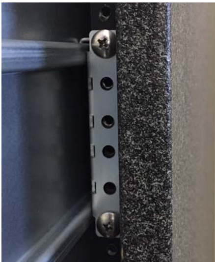
Figure 6. Aligning Inner and Outer Rack Supports
